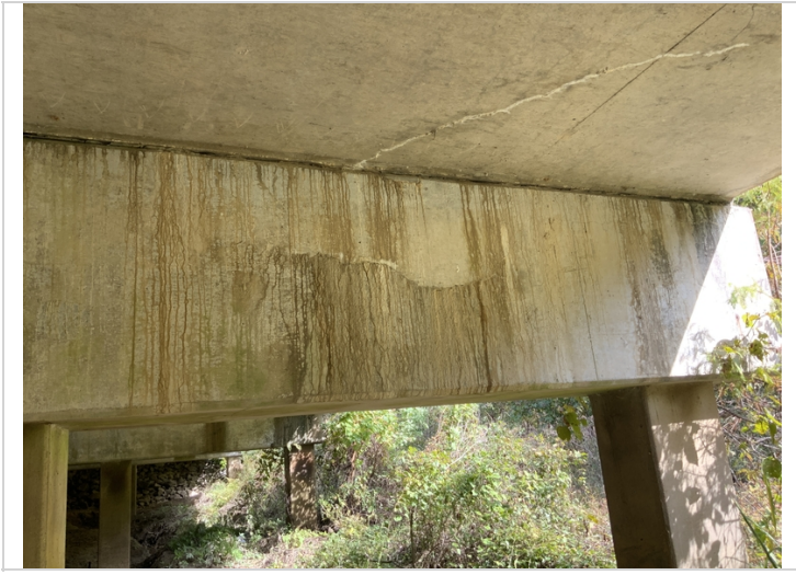
Bent 5 cap back, crack right end.
