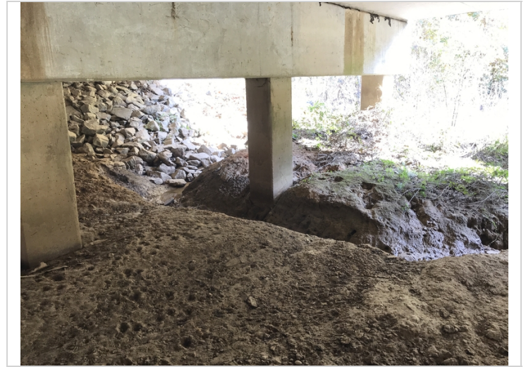
Span 7 looking ahead & Rt. @ scour hole running from outside Rt. & between piles 6 & 7. This is a drainage ditch than runs from bent 5 to ahead of bent 7.
