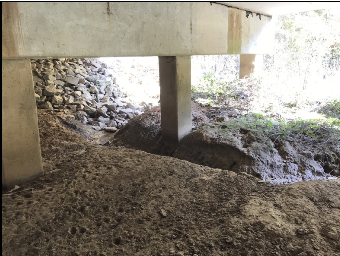
Span 7 looking ahead & Rt. @ scour hole running from outside Rt. & between piles 6 & 7. This is a drainage ditch than runs from bent 5 to ahead of bent 7.
