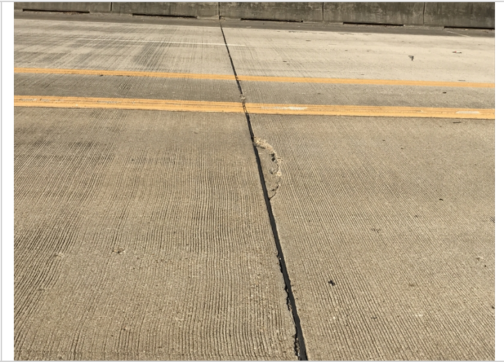
Span 4 @ bent 4 Rt. Inside Main Lane 4' Rt. Of C/L there is a large crack & small spall @ the joint.
