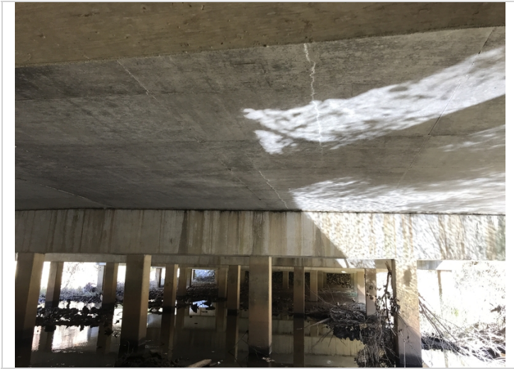
Span 2 looking ahead from bent 2 @ deck soffit cracks with efflorescence.
