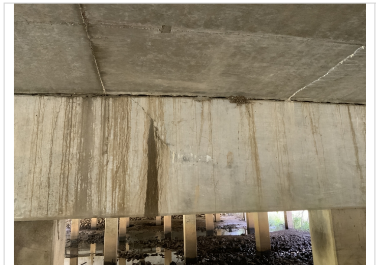
Bent 5 ahead, crack between piles 4 and 5
