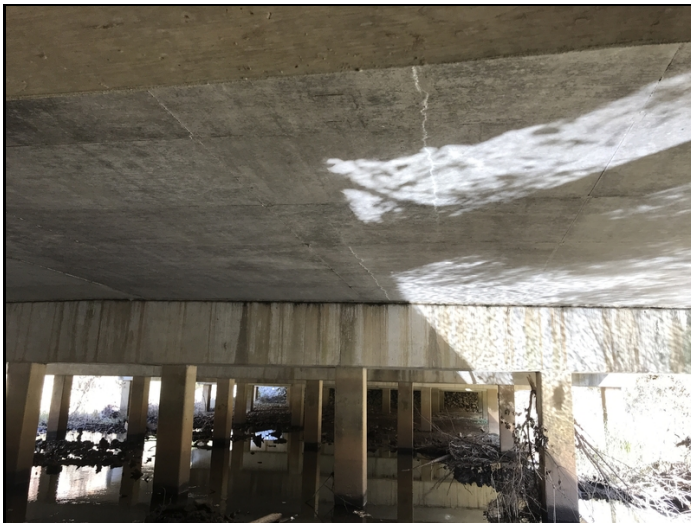
Span 2 looking ahead from bent 2 @ deck soffit cracks with efflorescence.
