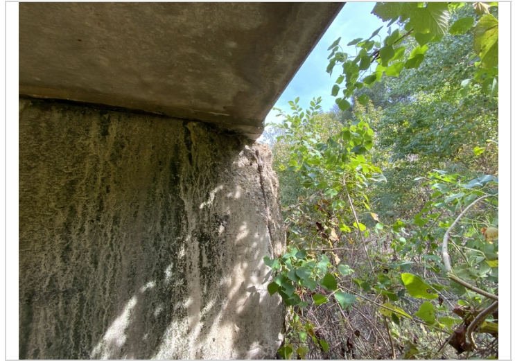
Bent 6 right end of cap spalled
