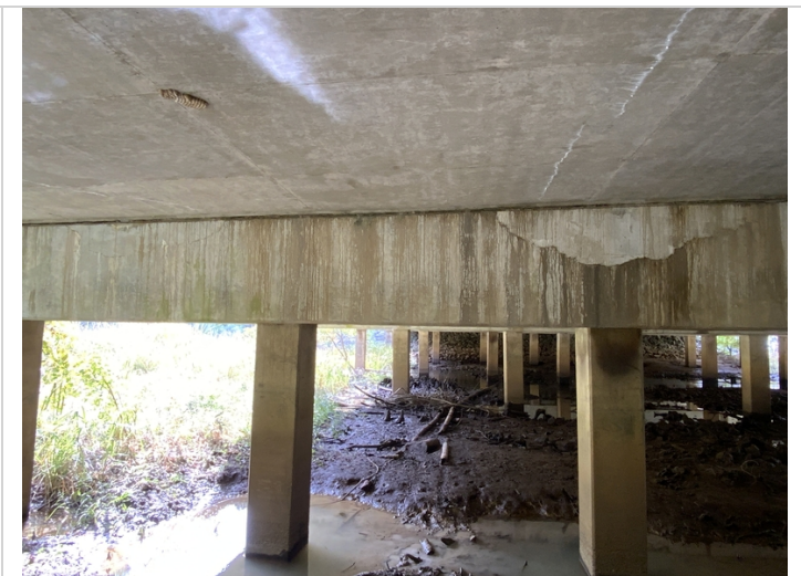
Bent 5 ahead, delams over piles 6 and 8
