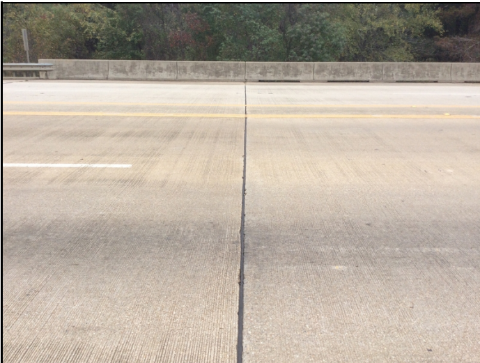
Joint material bent 2, is worn & tattered and is losing bond with the concrete. This is typical of all joints.
